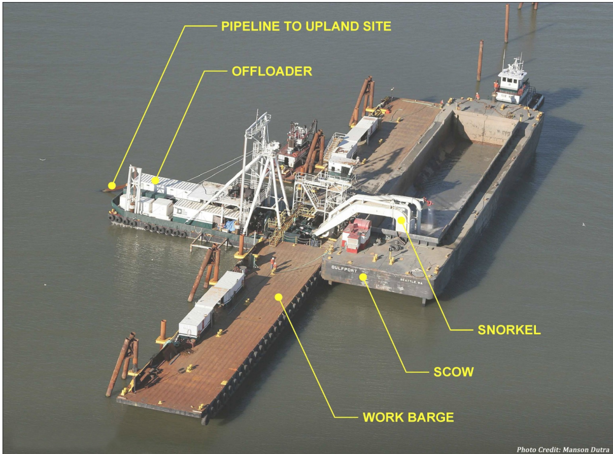
Figure 5-3. MWRP Offloader (Liberty) Unloading Scow
